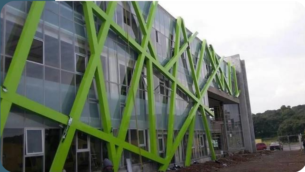
Hotel Autopista Mex- Qro Supply & installation of aluminum panel.
