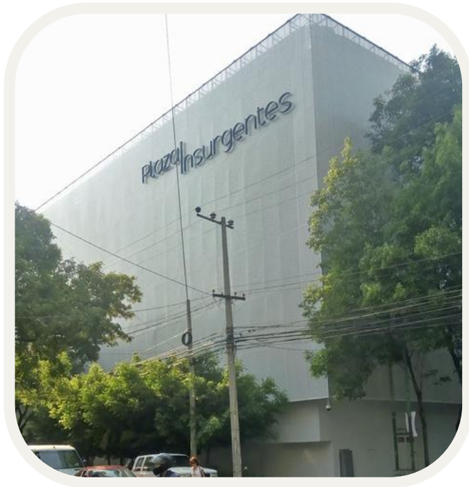
Plaza Insurgentes Supply and installation of multiperforated sheet.
